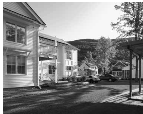
VERMONT INTEGRATED ARCHITECTURE
